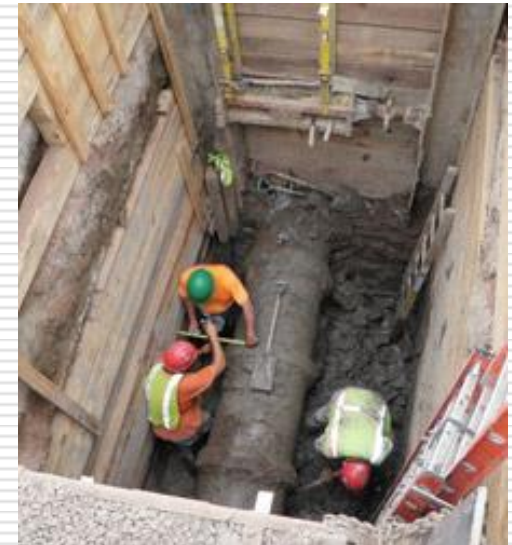
MDC Clean Water Project Excavation
