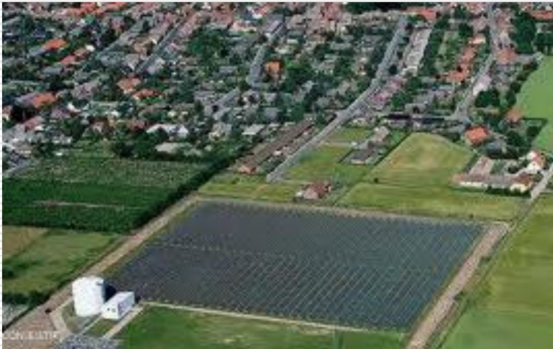
Marstal, Denmark 1,500 Customer Solar District Energy Solar Thermal Provides 50% of Space Heating Integrated Solar, Heat Pump and Biomass Boiler/ORC Fueled on Locally Produced Biomass
